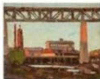
Trestle at Parry Sound TT-221
